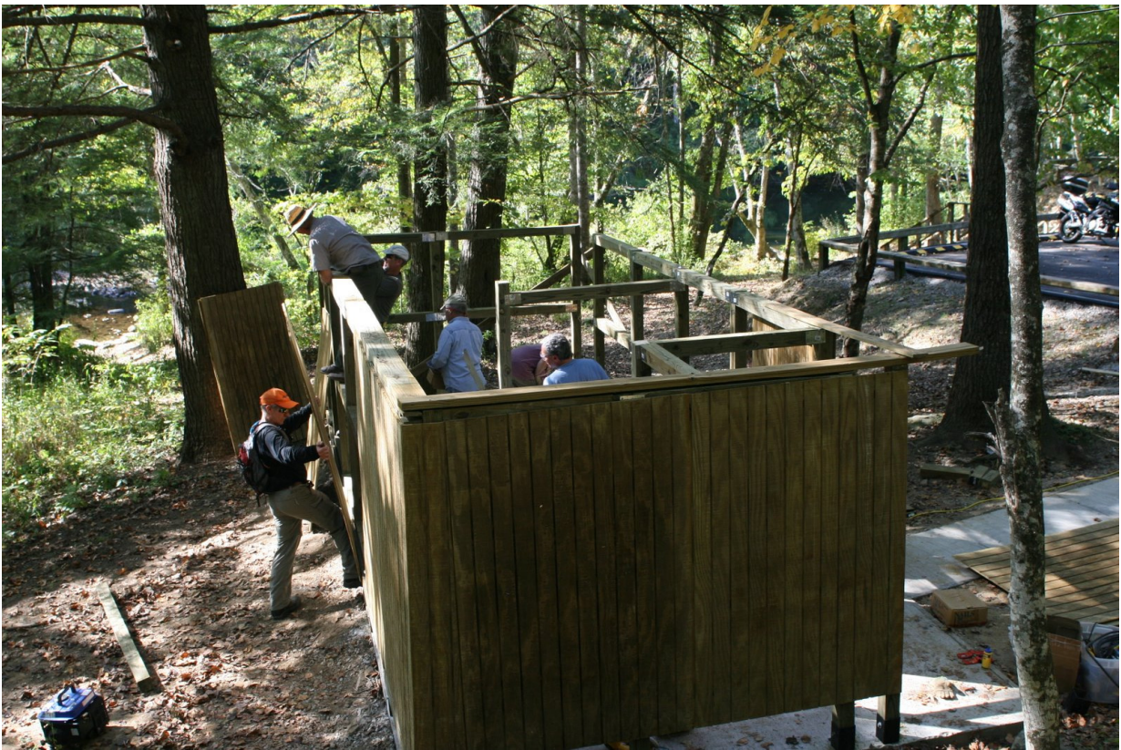
Change house begins to take shape.
